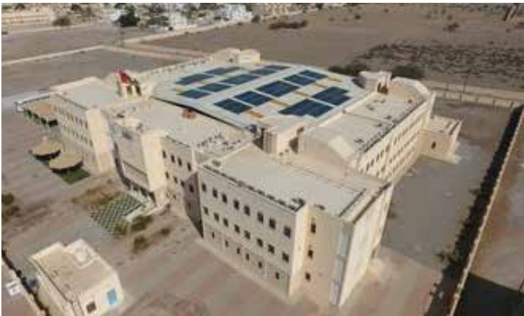
Picture of roof-top PV solar project installed at the school in Barka.
